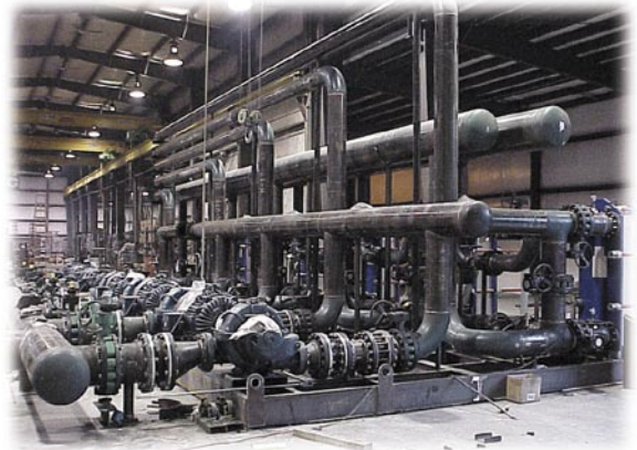
Mill System Pump Base Under Construction
