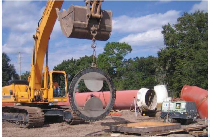
*The thin profile of the Westfall Model 2800 mixer makes it feasible to air ship anywhere in the world. The short laying length is a fraction of traditional mixers, making it less costly to produce, ship, install and maintain.*
