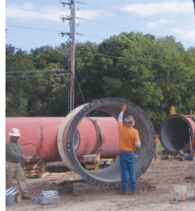
*72" diameter Westfall Model 2800 mixer, shipped with integral gasket and pre-drilled flange, requiring less heavy equipment for installation.*
